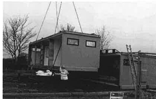
New Headquarters under construction
