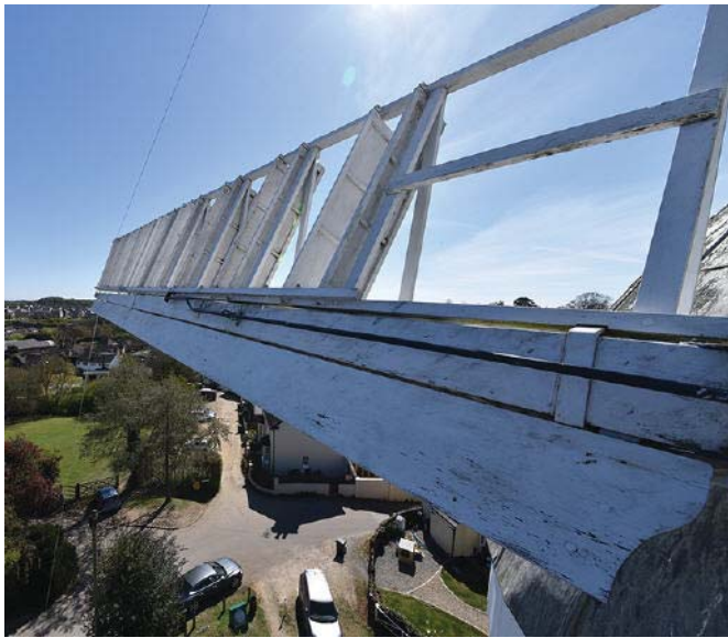
Restoration work has seen 20 panels refitted to the windmill's sails. Photograph Luke Thomas
