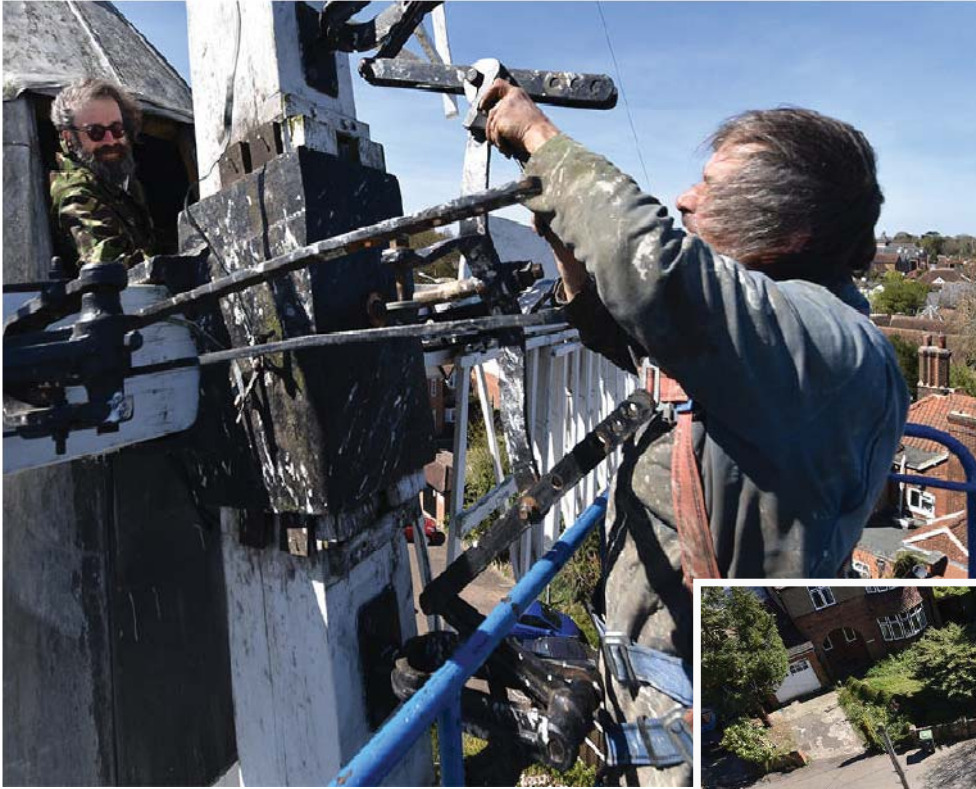
Tudor Owen, chairman of the Stansted Millers, looks out of the storm hatch while mill wright Paul Kemp carries out repairs to the windmill's striking gear 57ft above the ground from a cherry picker. Photographs Luke Thomas
